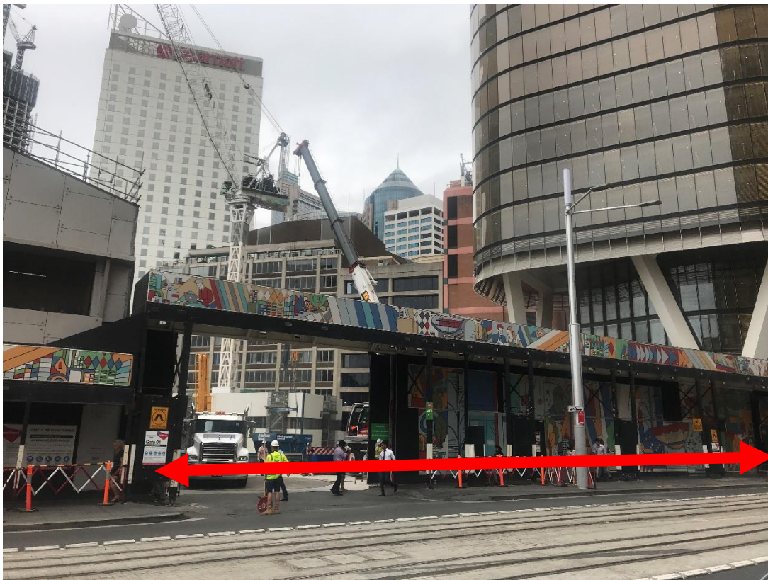
Figure 4: Site viewed from George Street
